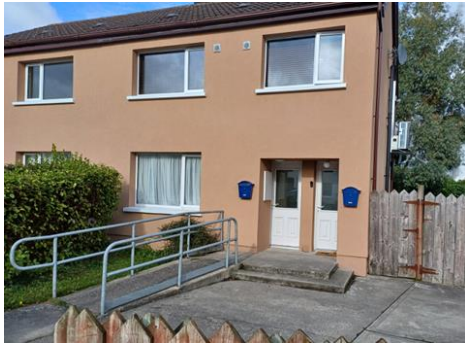
Monastery Grove retrofit upgrade.
